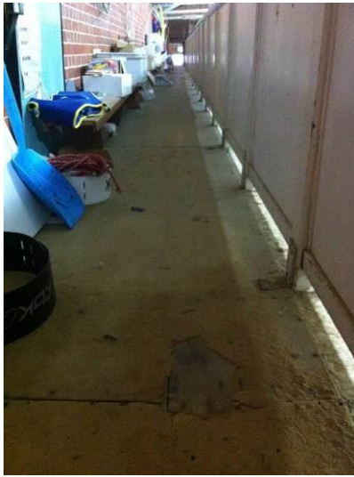
Floor covering to gallery on poolside
