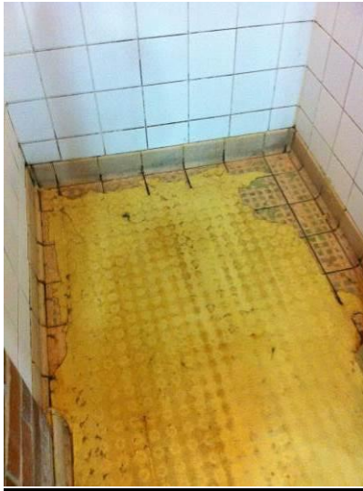
Eroded waterproof coating to shower area
